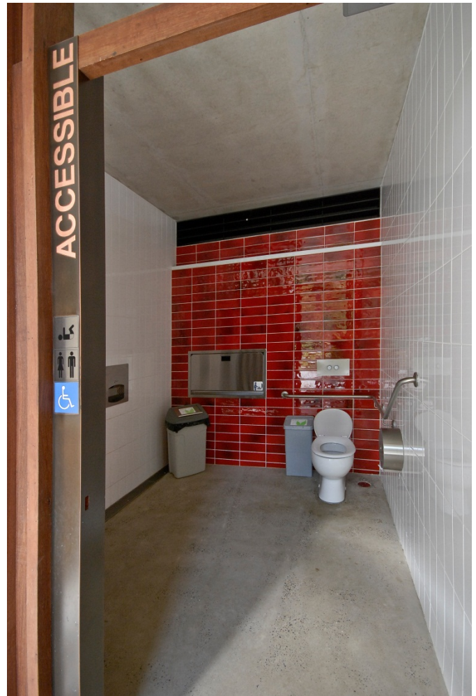
Pirrama Park toilets illustrating good practice inclusive access, large internal circulation space, and inclusive fittings and fixtures.
