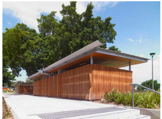
New toilet facilities at Turruwul Park, Rosebery
